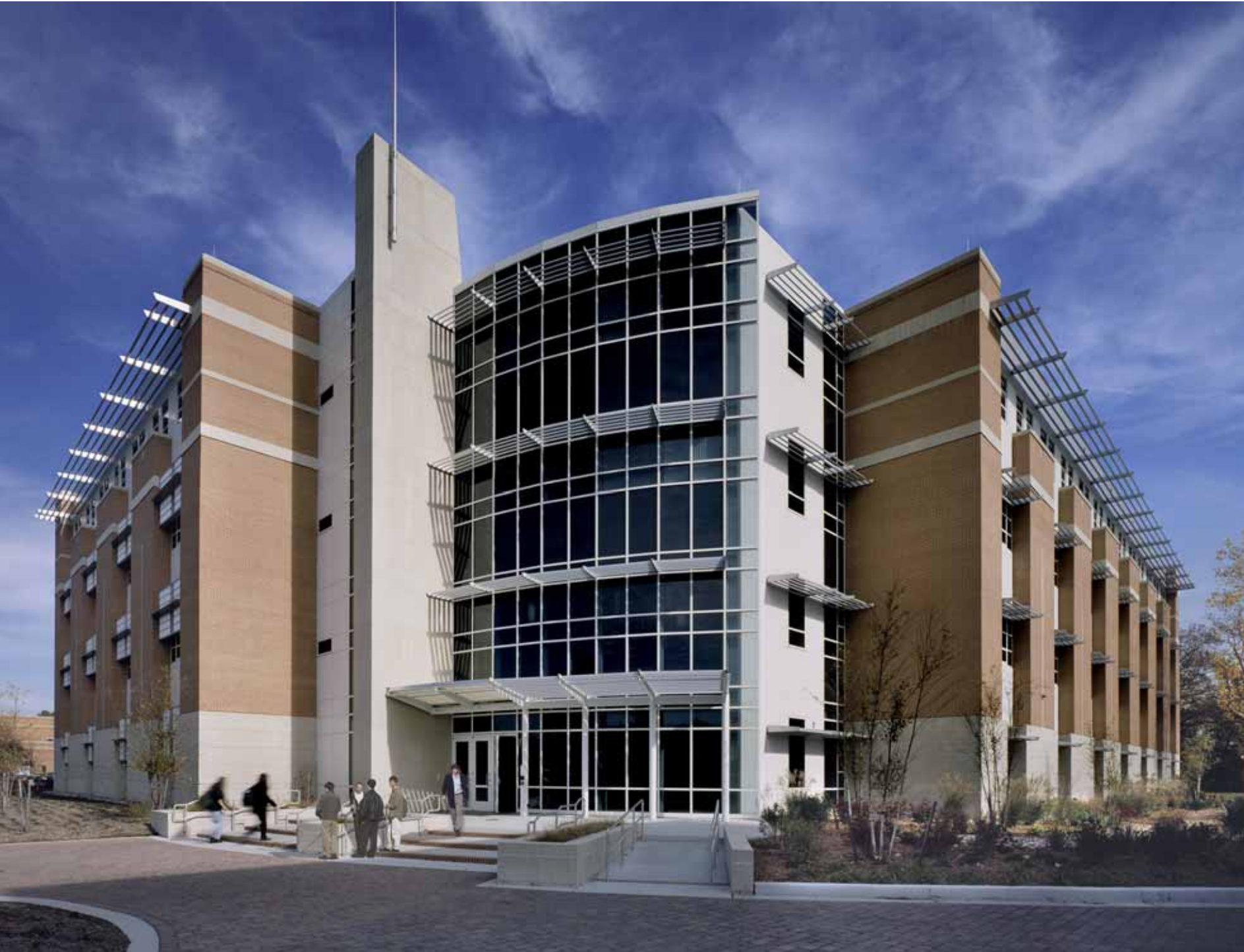
Exterior sunshades reduce heat gain, diffuse daylight, and unify the facade (left and right).
